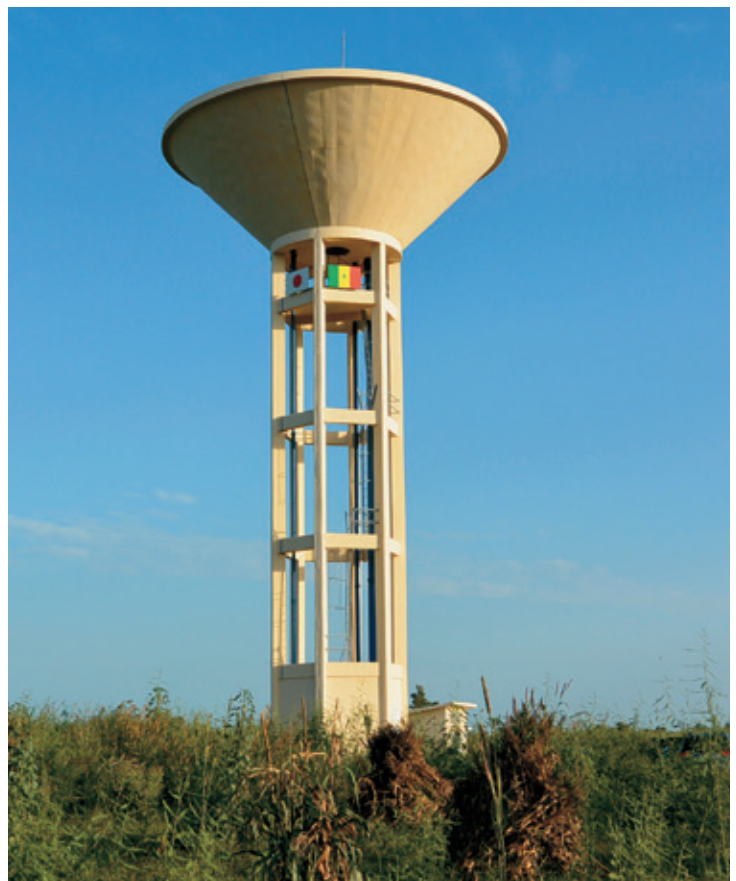
セネガルの青い空に映える高架水槽 / Elevated water tanks glowing in the blue sky of Senegal
